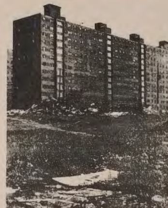
Mass vacant lots and physical deterioration of projects like Scudder Homes are reasons Newark housing is the worst in the USA.
