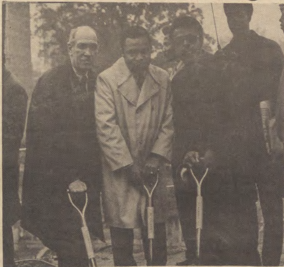
A Black Development! Groundbreaking for the 210 unit development of Kawaida Towers is focused on Counsel to Kawaida Towers, Raymond Brown, Mayor Kenneth Gibson and Imamu Baraka.
