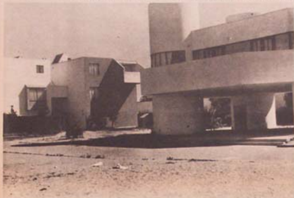
Acorn housing projects are becoming serious health hazards as rapid deterioration sets in. A corner of the project shown above.
