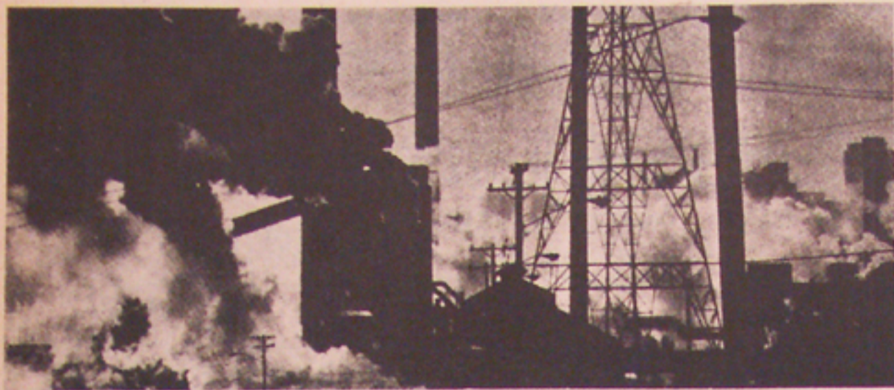
Pollution caused by U.S. oil refineries in Puerto Rico.
